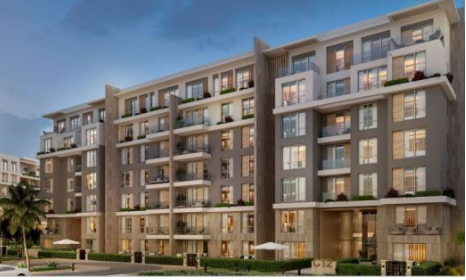
Building Type 3 - Front View
