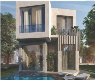
VILLA (C) // BACK FACADE
