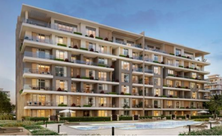
Building Type 3 - Back view
