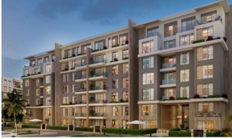
Building Type 3 - Front view
